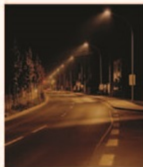
HPS 150W Insufficient light = Unsafe
